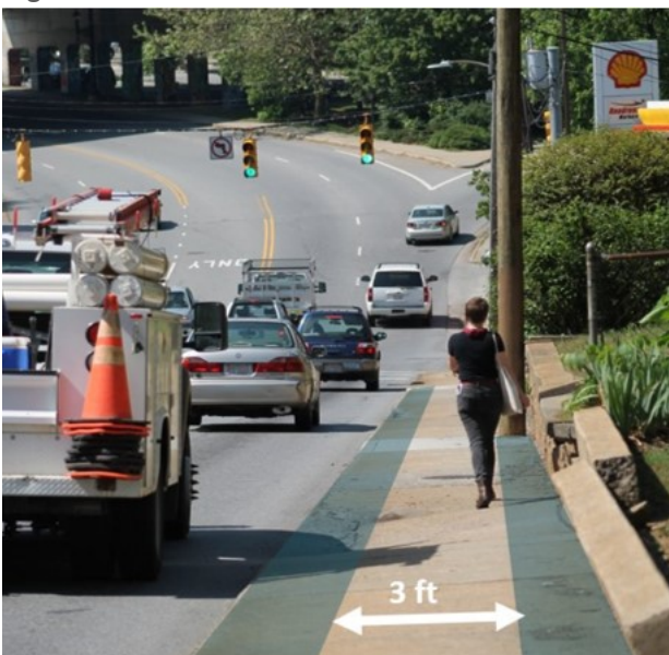
Figure 30: Effective Width of Merrimon Sidewalk
