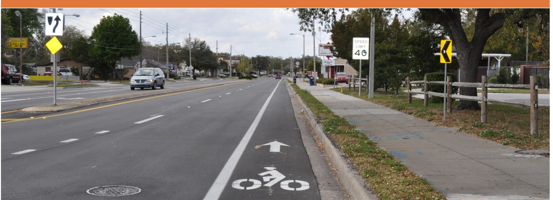
**Segment to the north (four divided & five lane) resurfaced with narrower lanes for bike lanes**
